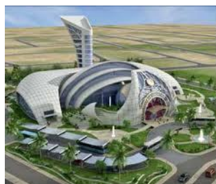
Figure 4 Kahrh Garden for Development, QSAS award for the Sustainable Building 2011.
